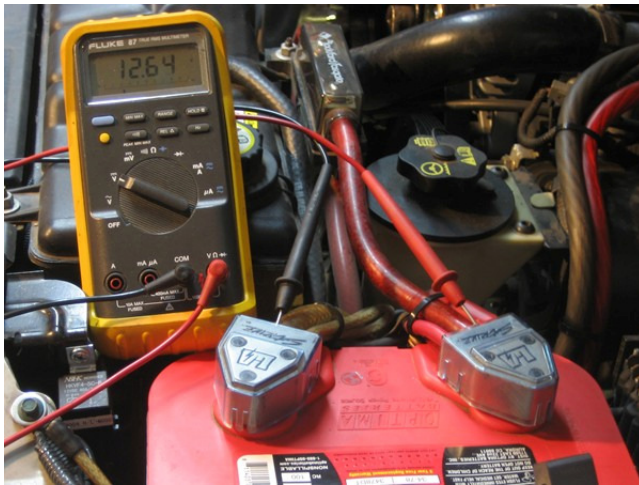
Standing voltage at the battery before starting should be in excess of 12.6 VDC. If not, see below.
