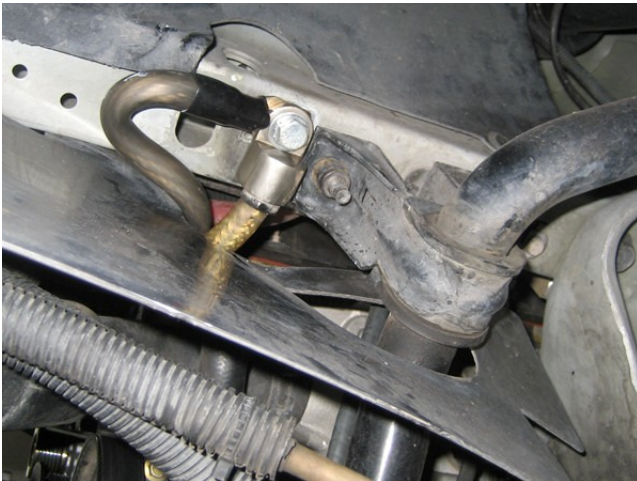
Connect the return path cables from the alternator and from the battery negative ( - ) to the subframe. Use star washers between the subframe and ring terminal, and between multiple ring terminals to ensure a low resistance connection. Tighten this bolt securely with a long handled ratchet. This step is VERY important!
